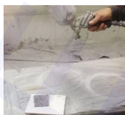
Figure 2: Application of the resin
